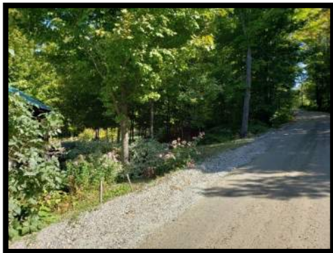
Photo B: Loose Shoulder Gravel
