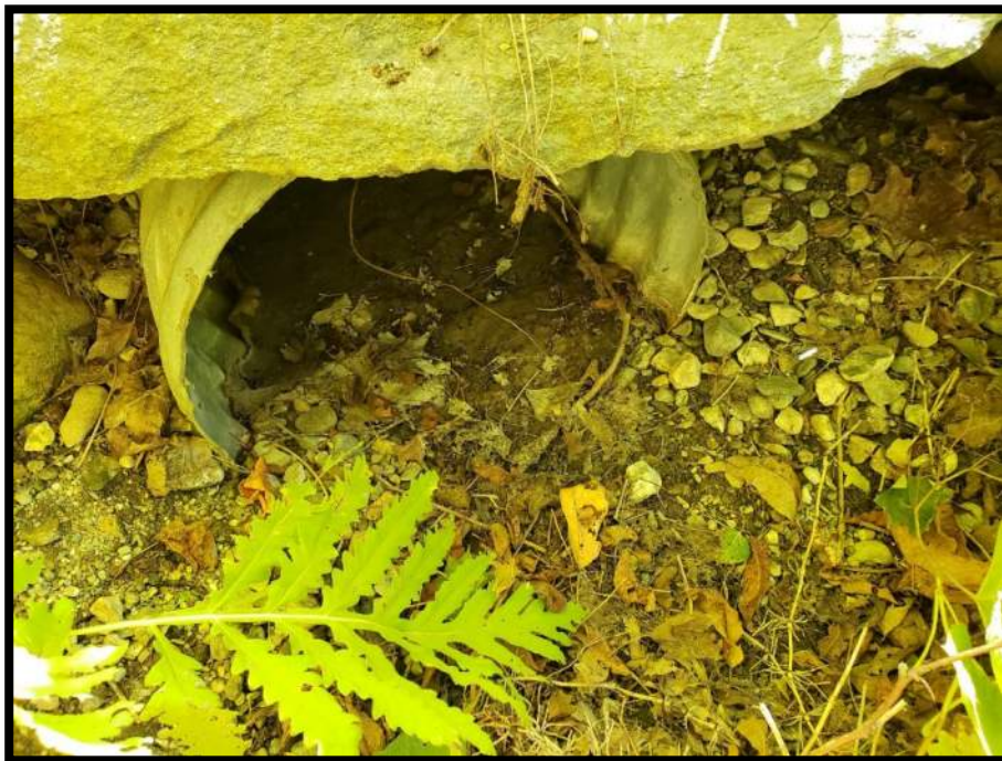
Outlet to an Existing CMP
