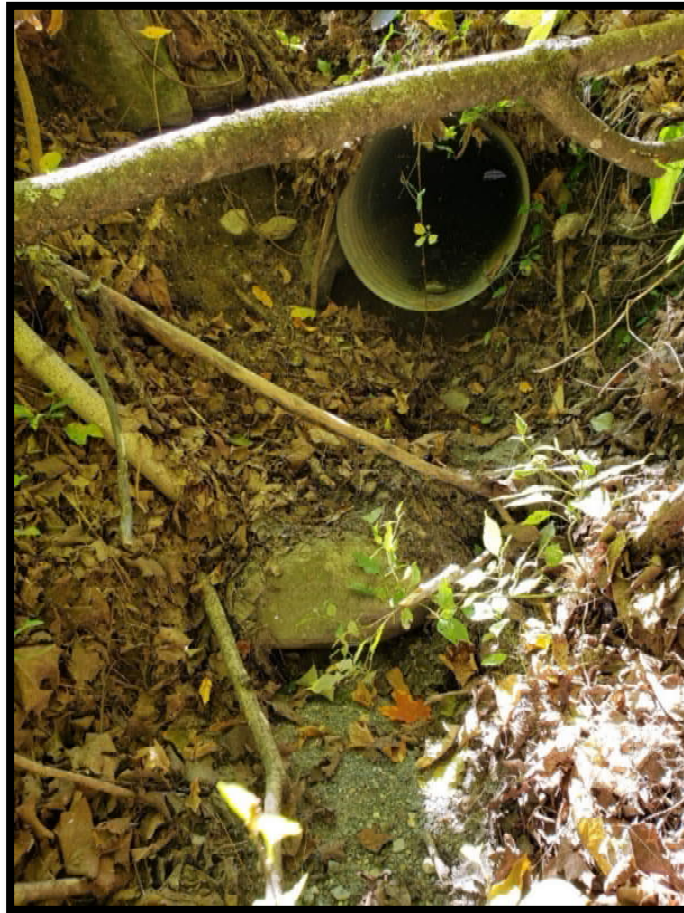
Eroded Outlet to an Existing CMP
