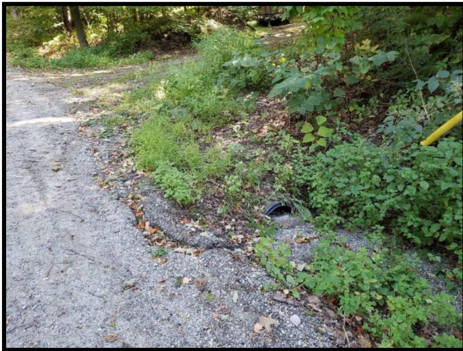
Drive Pipe and Rilling along Shoulder
